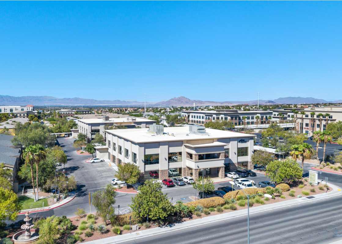
Covered entry and stone facade – the shared front door for 2900
